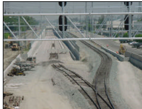
Overview of the entrance to the trench from a bridge above.
